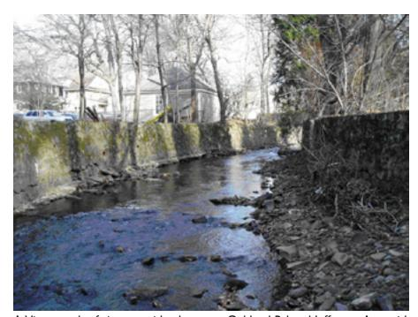
A. View north of river corridor between Oakland Rd and Jefferson Ave. with hand laid vertical stone retaining walls. Study area is characterized by State open waters and no areas of wetland. River bed appears to be scoured to bedrock with some cobbles on surface.
