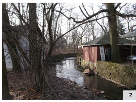
The river channel has stone walls with flat slopes along the residential west side and varying vegetated slopes along a majority of the east side. The wall is showing severe signs of undermining due to age and frequent storm events. River access would be difficult due to private property and tight conditions.
