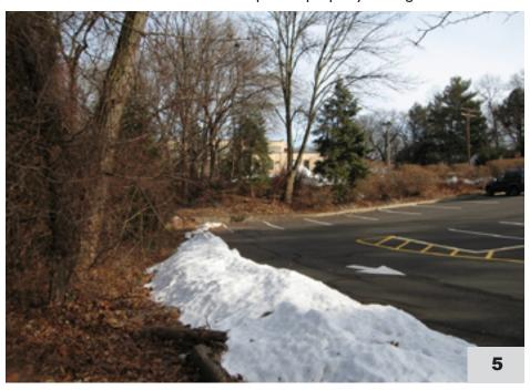
The lower Map Building parking lot is draining directly into the river and causing erosion on the slopes between the pavement on the wall. Consideration should be given to removing 25 feet of pavement and creating a rain garden to absorb surface drainage and clean hydrocarbons before the enter the river.
