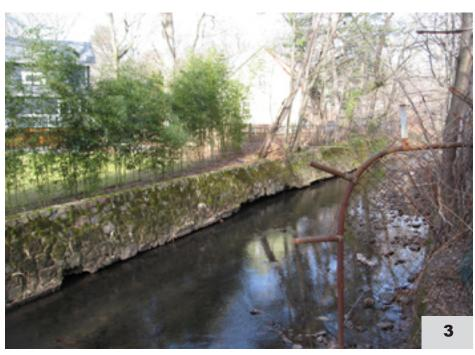
The river channel has stone walls with flat slopes along the residential west side and varying vegetated slopes along a majority of the east side. The wall is showing severe signs of undermining due to age and frequent storm events.
