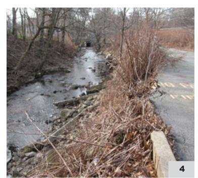
In several locations along the river the slope is severely eroded and in some cases failing making it unsafe. Reducing the paving width and returning space back to the river side slopes with improve safety, reduce erosion and increase access.
