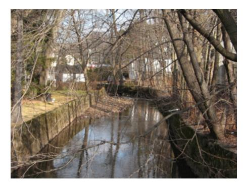
A. The river banks on the southern end of the project consist of hand-laid stone rubble retaining walls, that appear to date back to the 1930s. These walls are approximately 6 to 8 feet in height and exhibit varying degrees of distress. Of significant concern along the walled sections is the cutting of the riverbed along the wall resulting in undermining of the foundations. In some areas, development, including structures, extend up to these walls.
